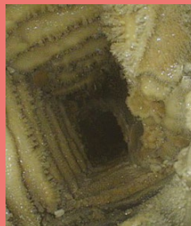
Figure 1.6 Cooling tower pack boroscope pictures
