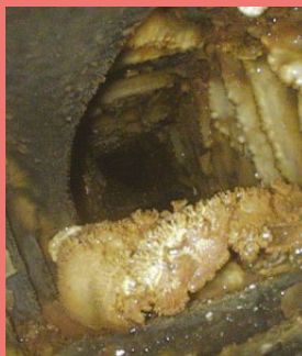
Figure 1.6 Cooling tower pack boroscope pictures
